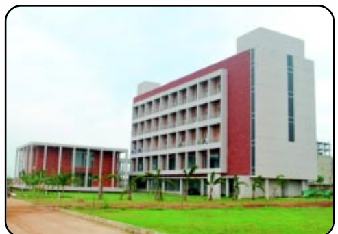
Outside view of the MDP Block
